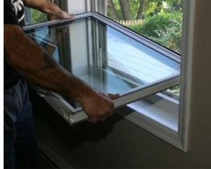
Hold the sash in a horizontal position and locate the sash tilt pins into the metal cams in the pivot shoes. Make certain they are engaged completely.
