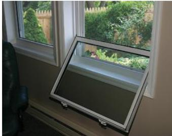
Raise the bottom sash up three inches above the sill. Using the tilt release latches at the top corners of the sash, push them towards the center of the sash and tilt the sash inward and allow it to rest on interior window sill. This will allow you to clean and it will not become disengaged from the pivot shoe.  *Holding the sash horizontally or parallel to the floor can allow the sash to come out of its pivot shoe while cleaning.*
