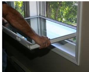
Once both tilt pins are in metal cams in the pivot shoe the sash should be level and horizontal. Using two hands tilt the sash upward into the operational position. Make sure both tilt release buttons on the top corners of the sash are completely engaged.
