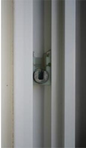
Using a regular straight screwdriver, turn the metal cam in the pivot shoe so the cam slot is horizontal or in the unlocked position. Using the screwdriver, position the left side 3 inches above the top of the sill and rotate the cam so the cam opening is at the top. This activates the brake and the shoe will remain in this position. Repeat on right side.
